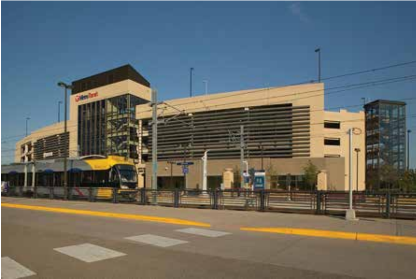
28th Avenue Park & Ride. ©Hanson Structural Precast 2013
